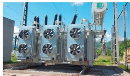
Auto-transformator montiran u TS Zenica 2
