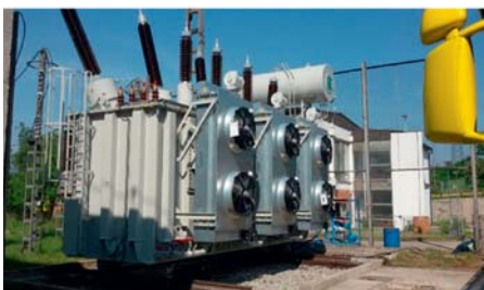
Auto-transformator montiran u TS Zenica 2
